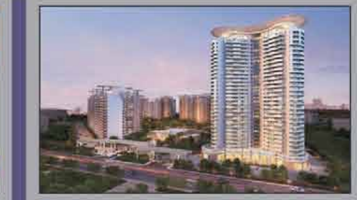
Park View Grand Spa Group Housing Complex. Located in Sector -81, Gurgaon. 3BR/4BR AC Premium Apartments. Total Apartments-694. Construction in Full Swing.
