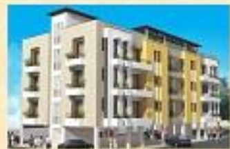
NOOR CITY 800, Street East End, Kharsa
