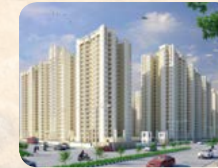
ATS ADVANTAGE PHASE II Indrapuram
