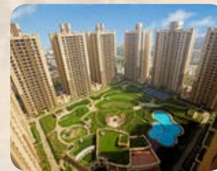
ATS ADVANTAGE PHASE I Indrapuram
